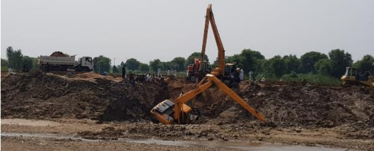
Filling of breaching point of Upper Jhelum Link Canal- UJC
