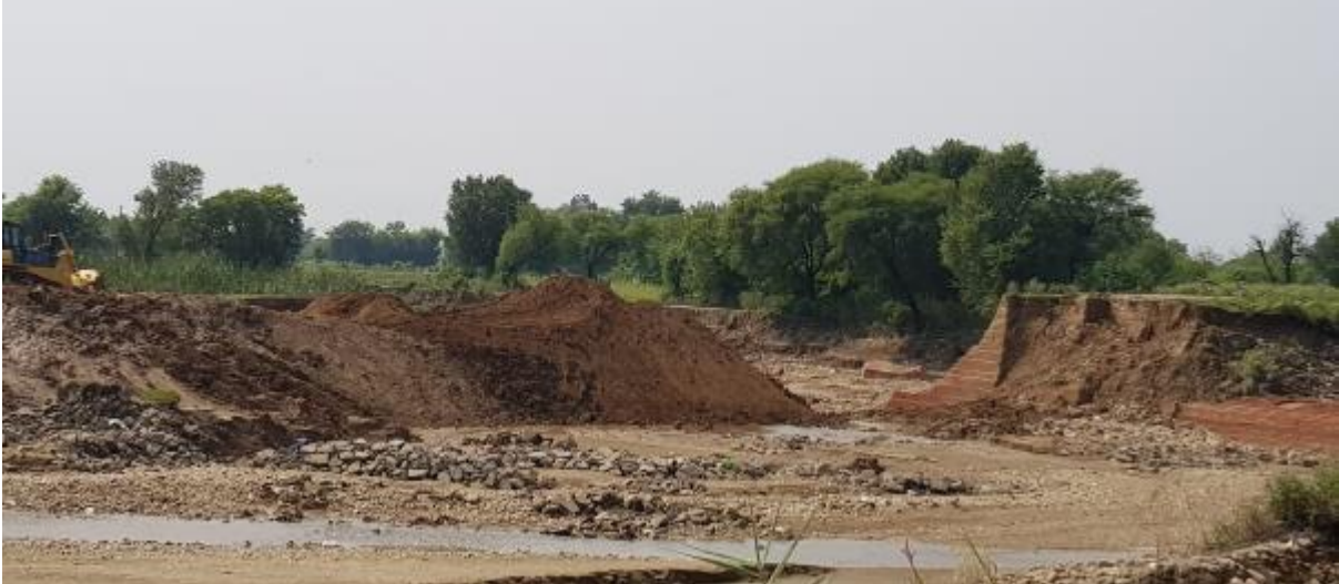
Filling of breaching point of Upper Jhelum Link Canal- UJC
